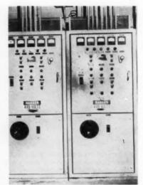
PRECIPITATOR CONTROL panels incorporate main power supply switch, voltage regulator, transformer start-stop buttons, rectifier-tube filament, rapper motors, high-voltage terminal heaters, and five voltage and ampere meters.
